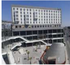
Ce Monterrey San Nicolás 2T22
